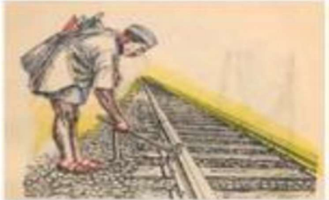
Figure 3: Manual Crack Detection By Human
